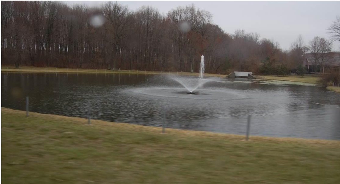
Figure A1-8. “Corporate Commons Pond” with gridwire exclusion system.
