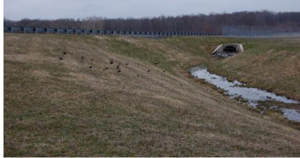
Figure A1-6. Drainage ditch near ANG Installation entrance.
