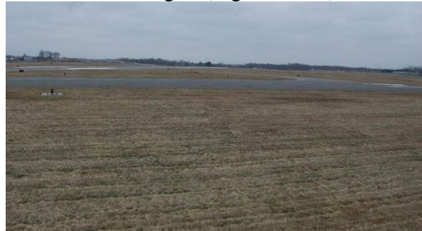
Figure A1-3. Airfield turf, well maintained.
