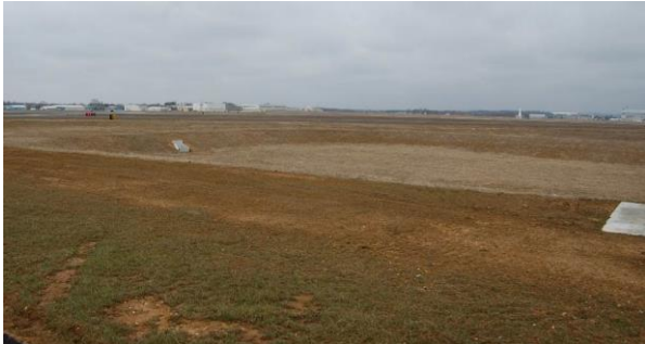
Figure A1-5. Newly constructed stormwater detention basin.
